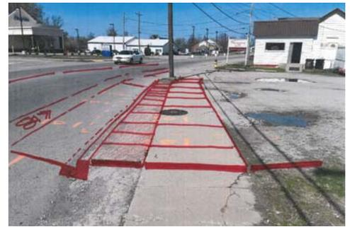
Figure 8: Sketch of proposed Sidewalk improvements on the east side of Spring Street near Harrison Street.
