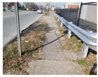
Deteriorating sidewalk and curb in the A&C segment
