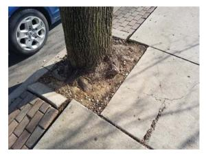
Tree roots causing damage to the sidewalk and curb-strip due to inadequate space
