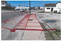
Figure 8: Sketch of proposed Sidewalk improvements on the east side of Spring Street near Harrison Street.
