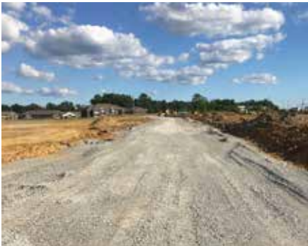
Access Road & Detention Construction
